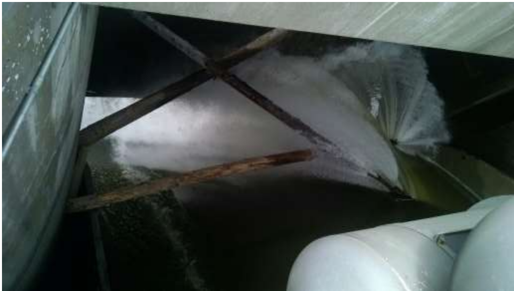
Photo 1. Logs across RSW prior to gate operation.
