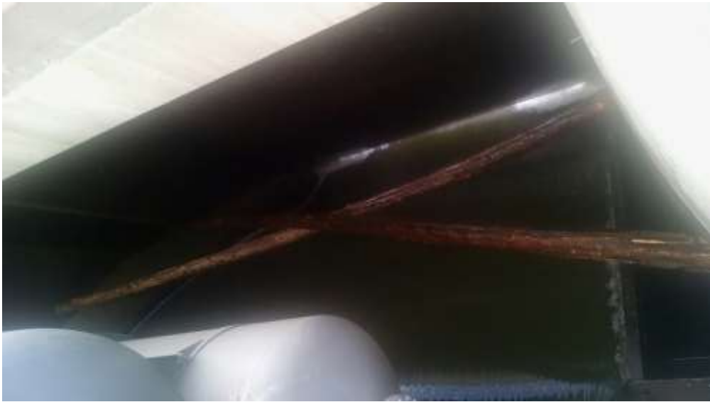
Photo 3. Logs across RSW during gate operation for log removal.
