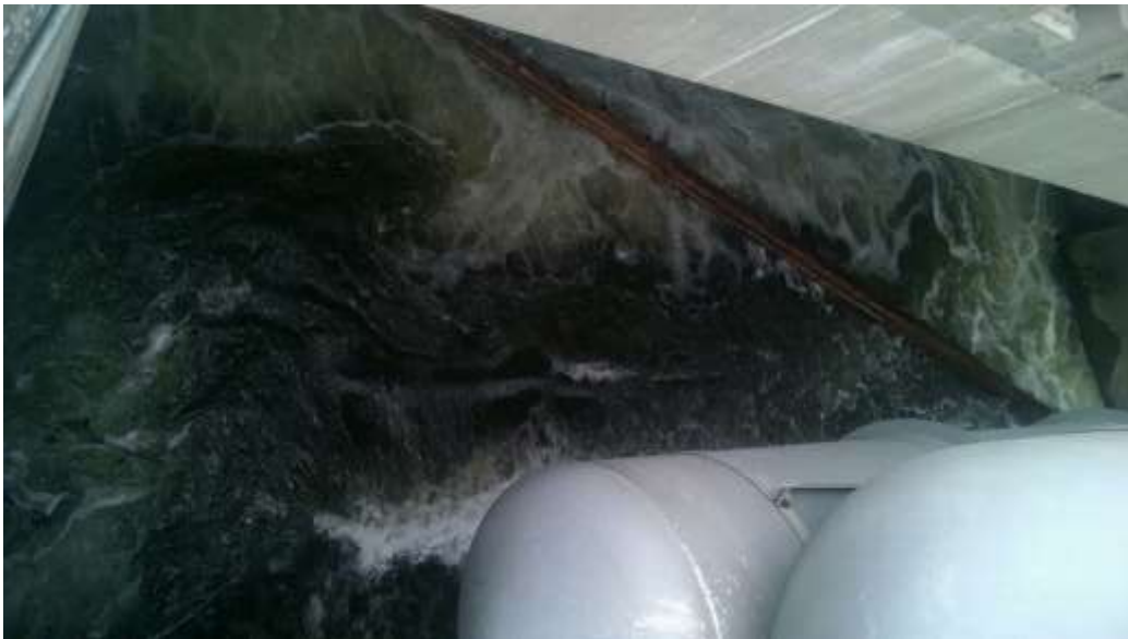
Photo 5. Logs across RSW during gate operation for log removal.
